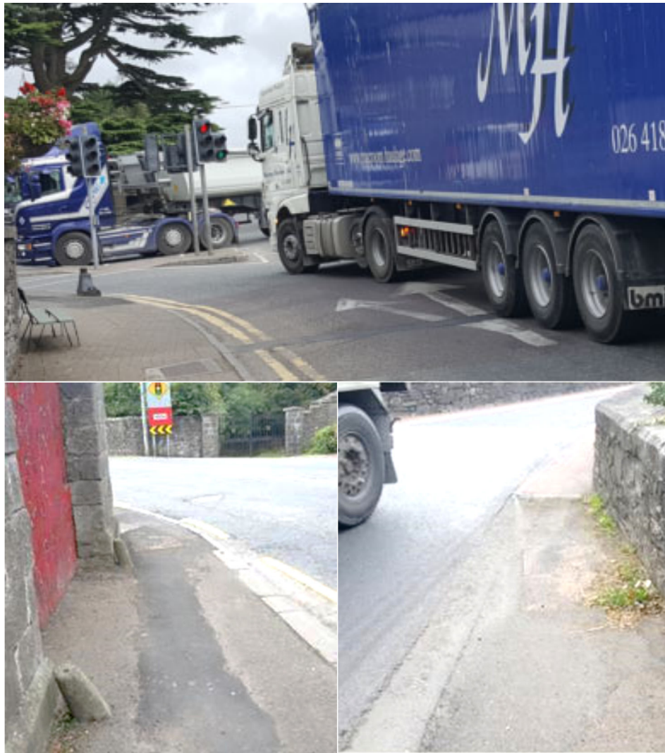
Figure 7.27: (Above) View of refuge island at the N2/N51 signalised junction in the context of turning HGVs; (Below) Examples of width restrictions on existing footways in Slane village
